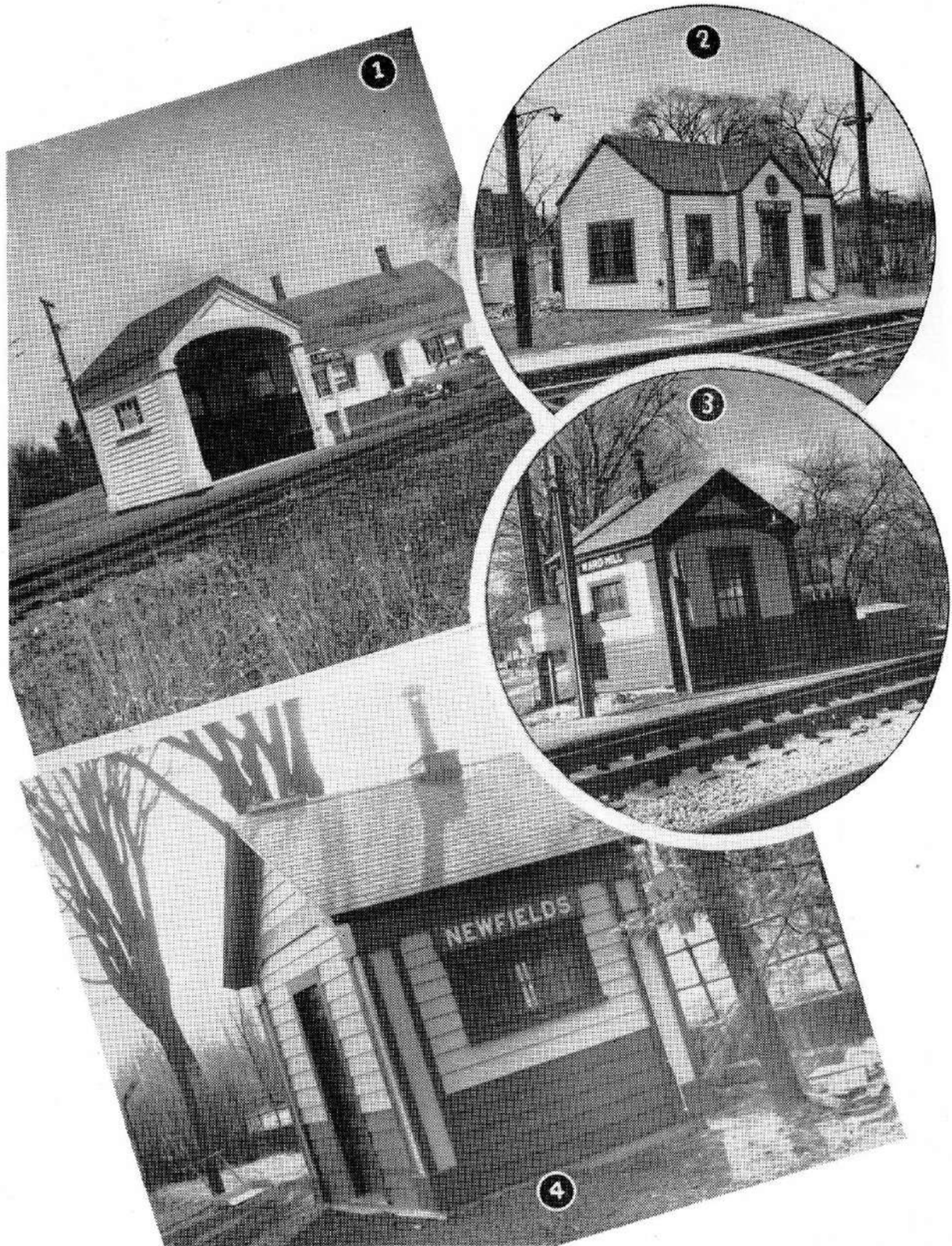
(1) Open front station at Lochmere, N. H. (2) Larger type, closed station, with stove heat, at Farm Hill, Mass. (3) Small, closed type station, with stove heat, at Ward Hill, Mass. (4) Station at Newfields, N. H., similar to that at Ward Hill
