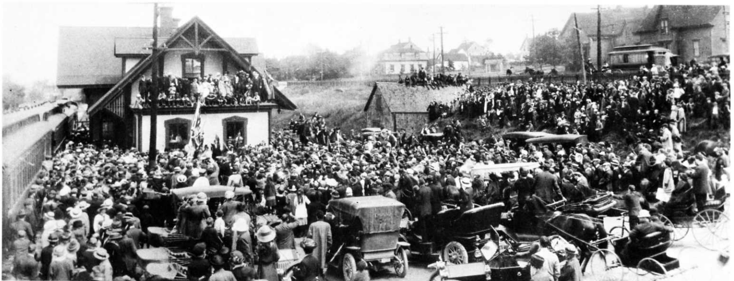
One of the ex-Washington cars appears at the extreme right in this view taken in 1917 or 1918 at the South Paris depot. Why the crowd? Undoubtedly future World War I Doughboys were being given a rousing farewell as they left for basic training.
