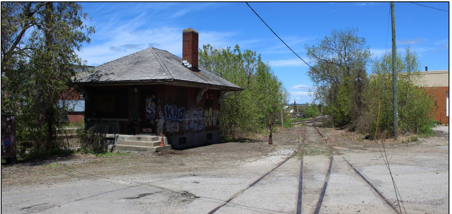
Below: A lot has. MA Tower, closed since 1974 and photographed nearly 75 years later on May 11, 2019. Union Station has been gone since 1962; the engine facility is now a ballfield; the Manchester segments of the Manchester & Lawrence and Portsmouth Branches have been silent since 1989. Only the mainline and a bit of the yard remain in service. The tower is soon to vanish. Rick Kfoury photo.
