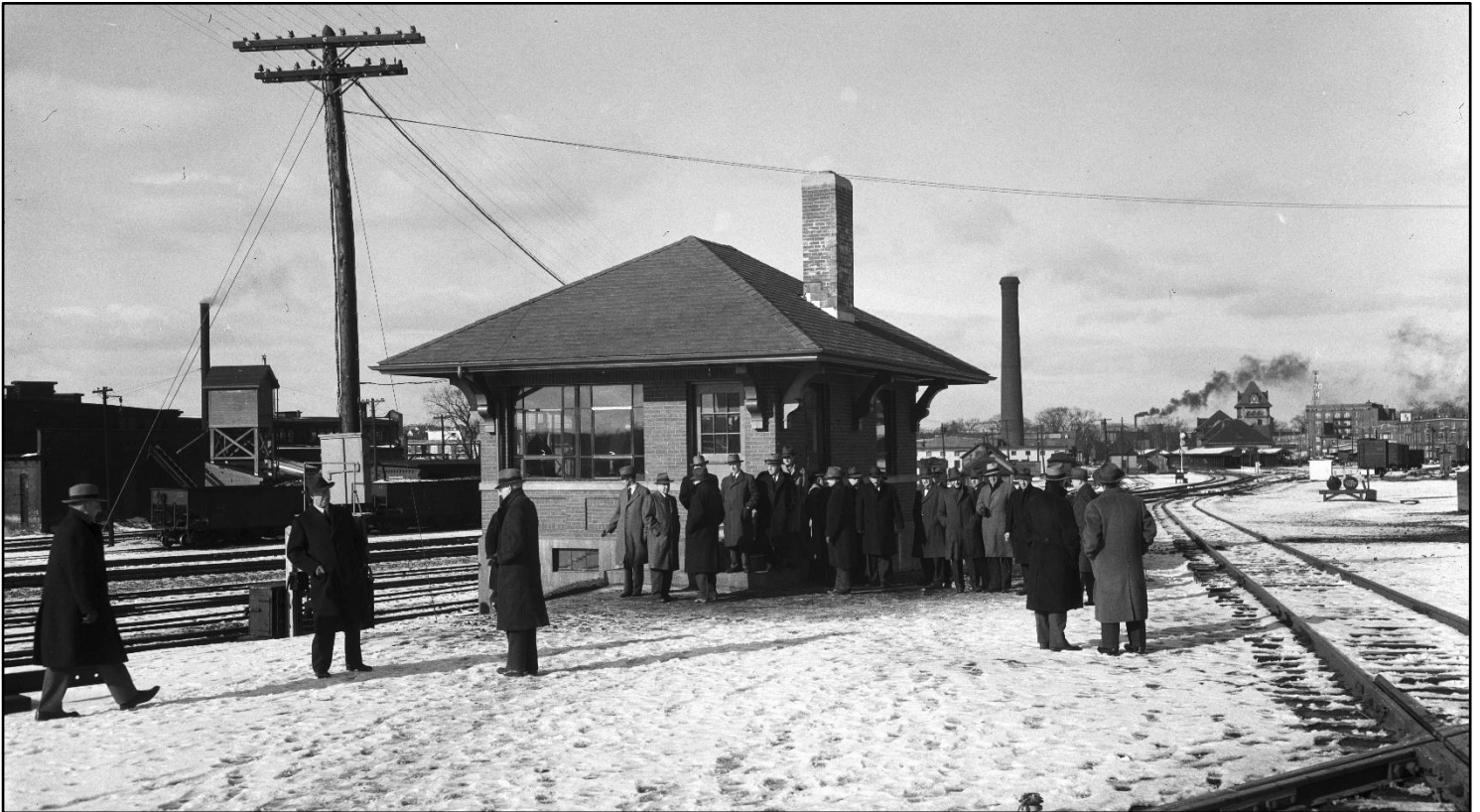
Above: The new CTC signal tower at Manchester (MA Tower) opens on December 13, 1944. Note at right the Manchester & Lawrence Branch and diamond crossing for the lead into Hill Yard. Union Station looms in the distance. How much has changed?
