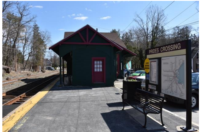
While Prides Crossing depot still proudly stands in its original location, a few modern MBTA commuter rail amenities have been added over the years to the location, such as modern signage and platform graphics. It is unclear what will become of these items with the end of passenger service. Andrew Riedl photo 3/27/2021.
