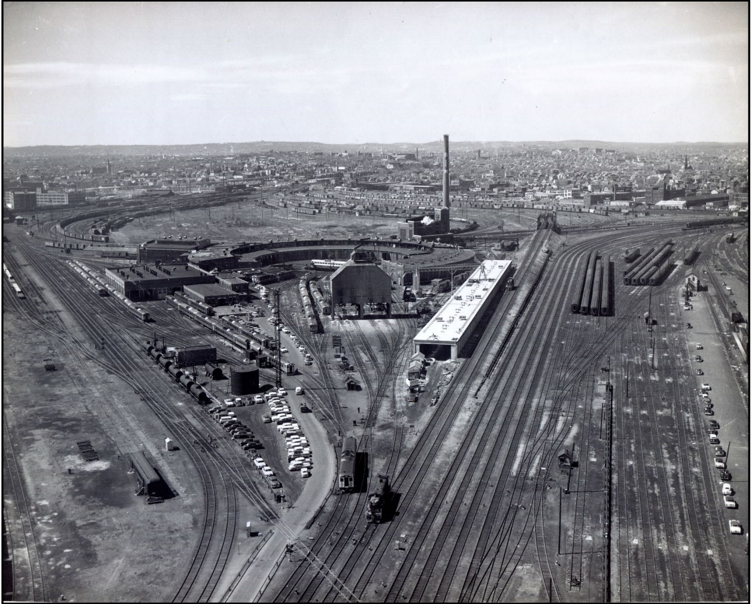
The Boston & Maine's Boston Engine Terminal and surrounding facilities at East Somerville, MA, circa 1957. Note the "Budd House" which has just been completed, is awaiting the installation of track.
