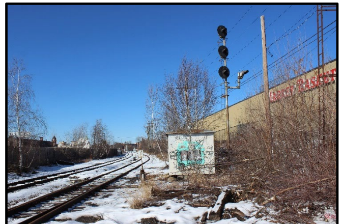
Above: Signal heads on the northbound signal at CPN 28 turned to face away from the mainline. February 19, 2020.
