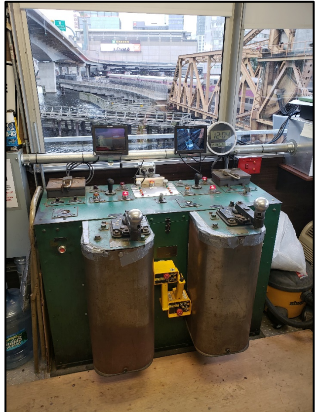
Clockwise from top: Old and new side by side; the control room in the new tower, featuring the same drawbridge controls from the old tower; the newly completed structure; and the old brick tower, which entered service November 13, 1931 and operated as an interlocking tower until 1993, when operations were consolidated to a new dispatch center at Cobble Hill in Somerville, MA. Until recently, only the drawbridges were operated from the old structure which awaits demolition.
