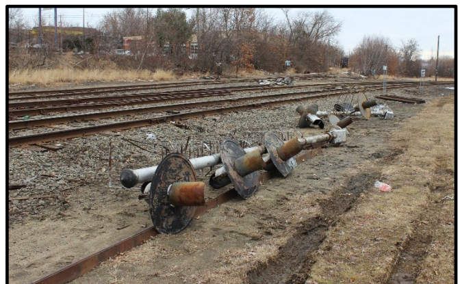
Below: Signals cut down and awaiting removal in Manchester Yard. February 26, 2020, Rick Kfoury photos.
