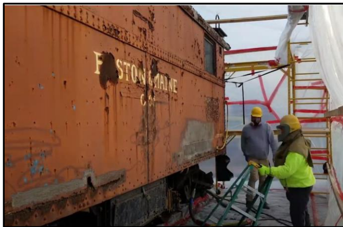
EnviroVantage workers begin sandblasting in early October. Beneath the Raymond Historical Society's last paint scheme can be seen original patches of blue and the B&M "McGinnis" logo from its service life on the Boston & Maine Railroad!
