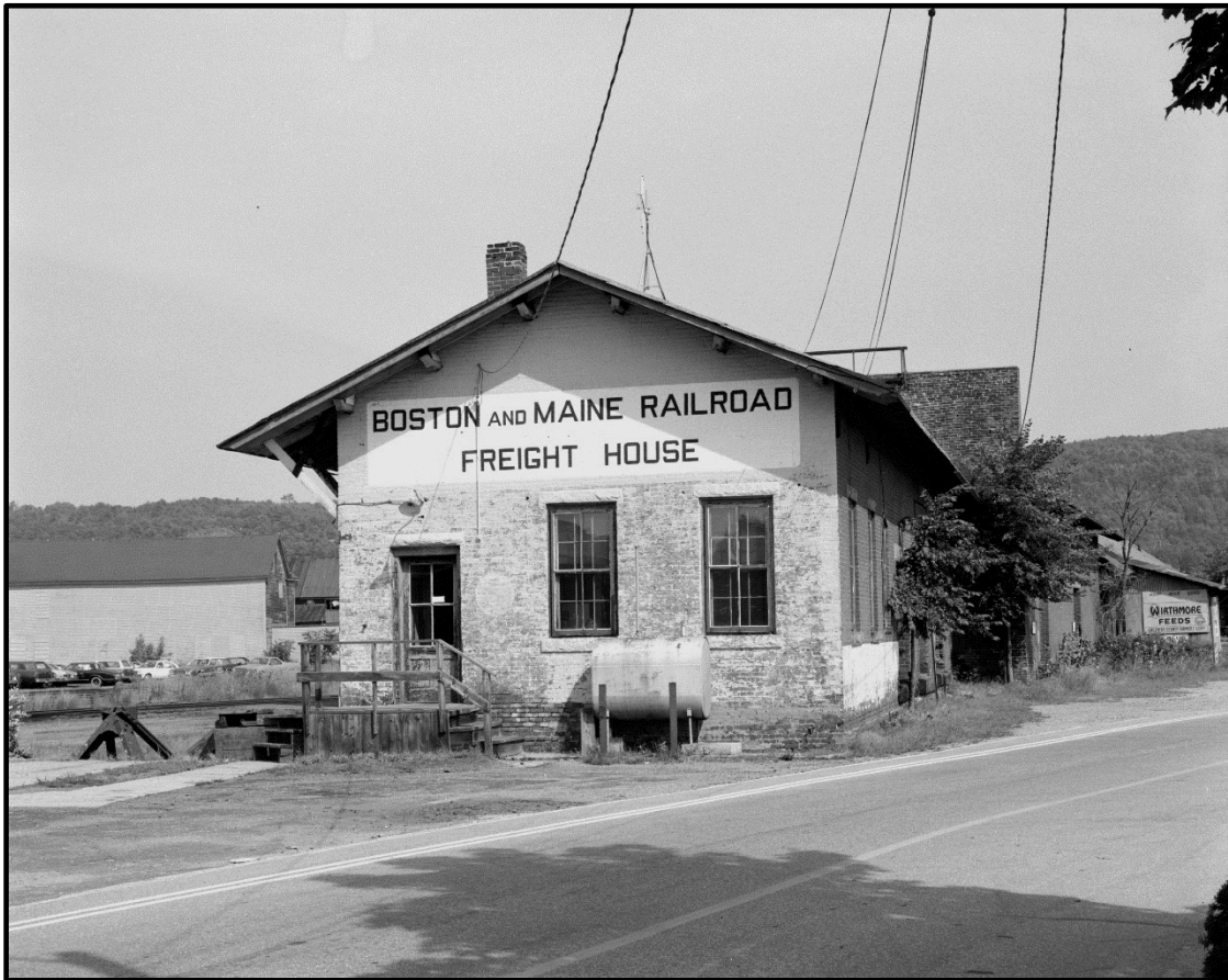
The B&M freight house at Keene, NH, September 1, 1979. Jack Armstrong negative, B&MRRHS Archives
