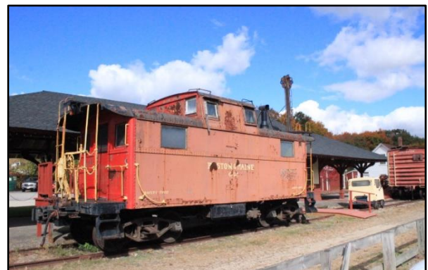
The station at Raymond, including N-5b caboose C-21 which is slated for repair and repaint. Rick Kfoury photo.
