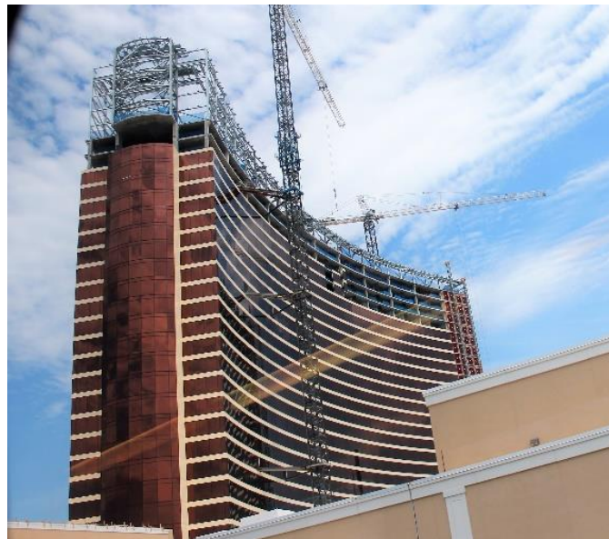
Casino under construction in Everett, Mass.
