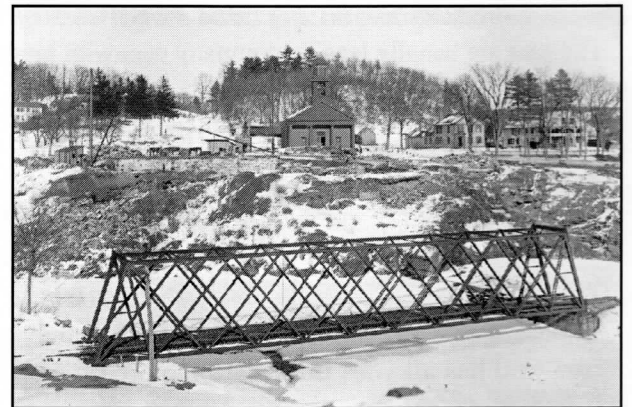
2/20/1904: A clear view of the old rail bridge, soon to be buried, as seen from atop the new causeway. Beyond is part of the former center of West Boylston, also soon to disappear.
