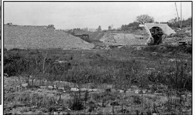
10/22/1904: Taken from the other side of the new causeway, looking northwest, this also shows the old bridge partially entombed, while the new arch bridge nears completion.
