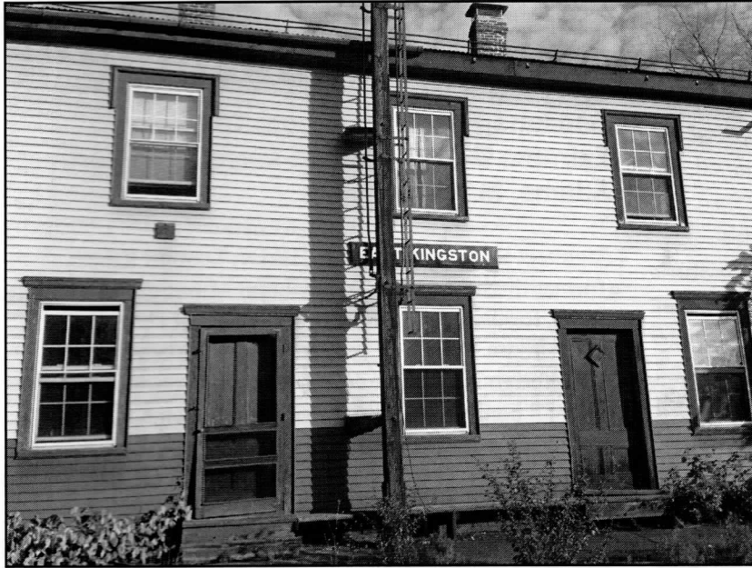
Trackside view of station
