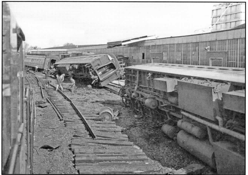
Appears B&M GP-7 early 1555 "class" on "southbound" NH Division mainline at "NUS", coaches on torn up "northbound" NH Div. mainline with surrounding team tracks of station and storage tracks that serviced the Johns-Mansville Gypsum (sheetrock) manufacturing plant. Note the missing passenger trucks on coaches. Johns-Mansville in those days offered their "gypsum" scrap products as "landfill" to contractors. Many of the local communities took advantage of free landfill.
