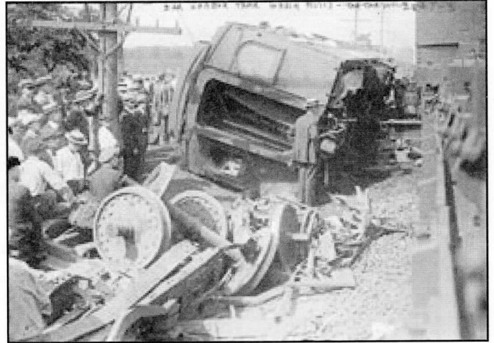
Townsmen and boys inspect the wreck of the Bar Harbor Express in Graniteville in this photo taken by Charles L. Hildreth.
