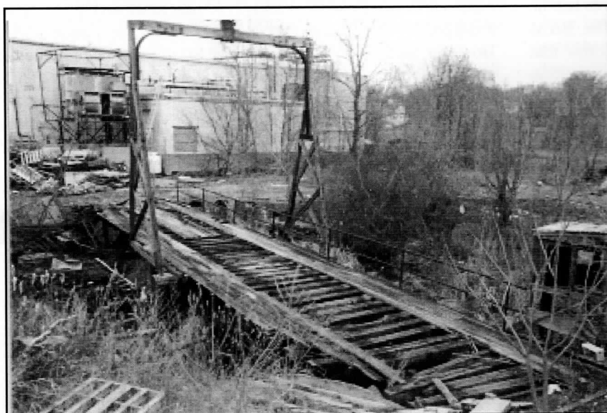
Looking West - despite the condition of the wood, the turntable is in excellent condition. There is still sand in the turntable cabin Traction ring hopper. The controller is missing.
