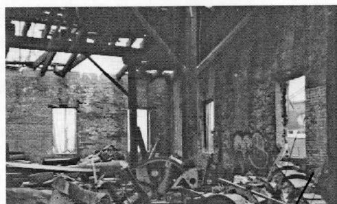
Looking northeast into Bay 1 Old highway plows and junk
