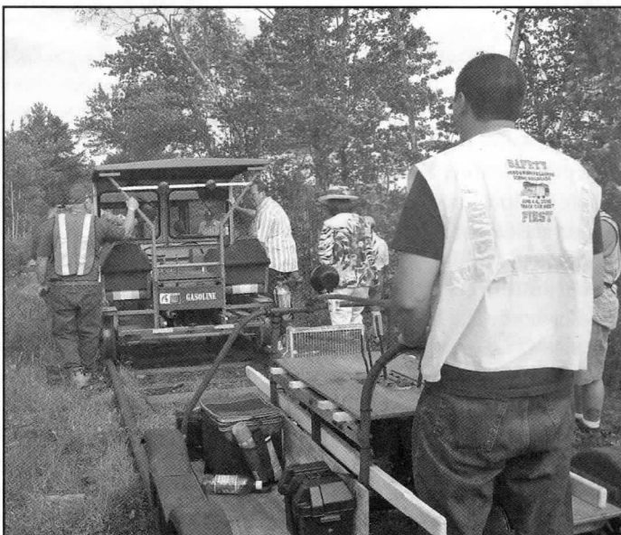
Getting ready to push over the slight new bridge.
