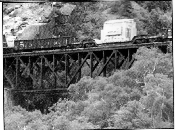
The consist crossing Willey Brook trestle
