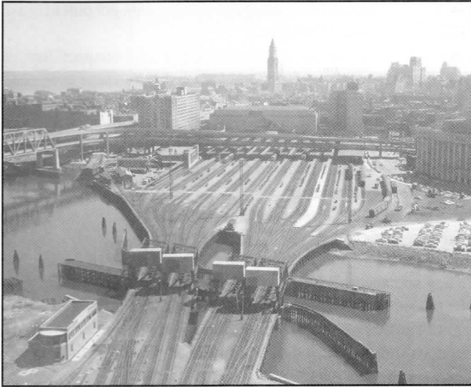
Aerial view of 1928 North Station looking south, 1957. Credit: B&MRRHS Archives.
