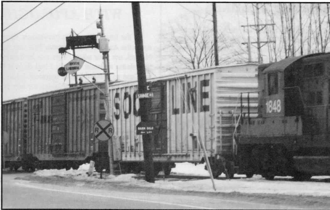
Last working Wig-Wag on the B&M at Jones Crossing, Rte. 101, Milford, N.H. B&M GP9 No. 1848 is pulling a local over the crossing in March, 1986. (B. Winiarz photo)
