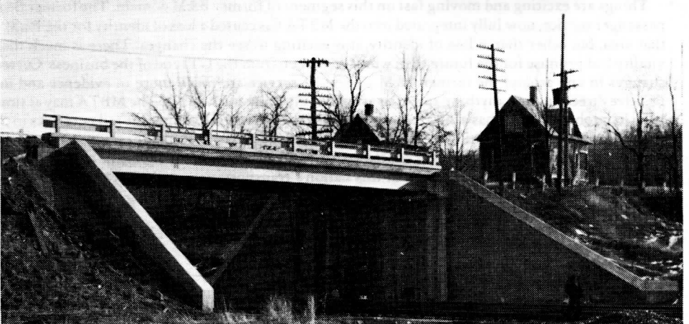
The new and the old at the west end of East Deerfield yards as an old covered highway bridge entering the yard is razed (top) and replaced by a new steel and concrete span as shown below
