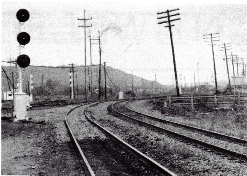
This photo from Arnold Greenleaf shows the "new" Boston & Maine/Delaware & Hudson interchange in Mechanicville, NY. You will notice that the Boston & Maine track in the foreground no longer crosses the Delaware & Hudson, but instead goes into the D&H yard.
