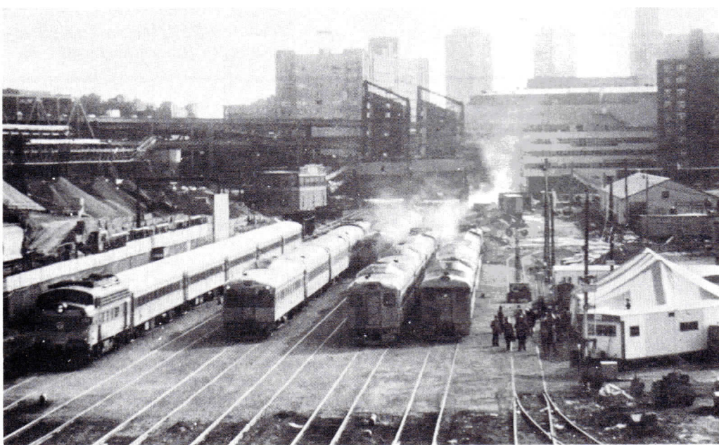
An overall view of the "interim" facility constructed by the MBTA after the North Station fire. This view from the old Prison Point bridge shows the filled-in yard tracks, and the temporary tent-shelter to the right of the tracks.
