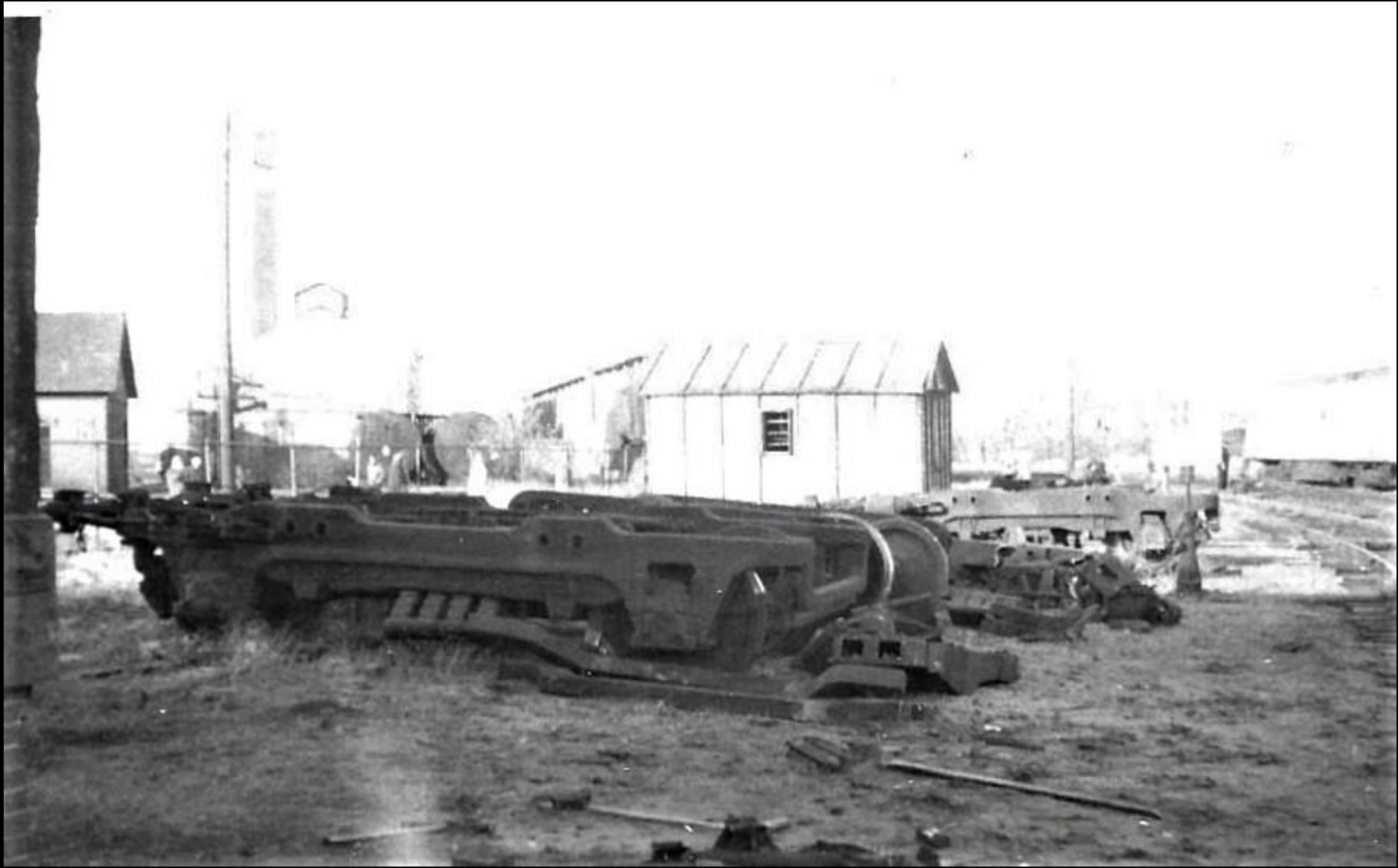
A Row of damaged derailed passenger Trucks
