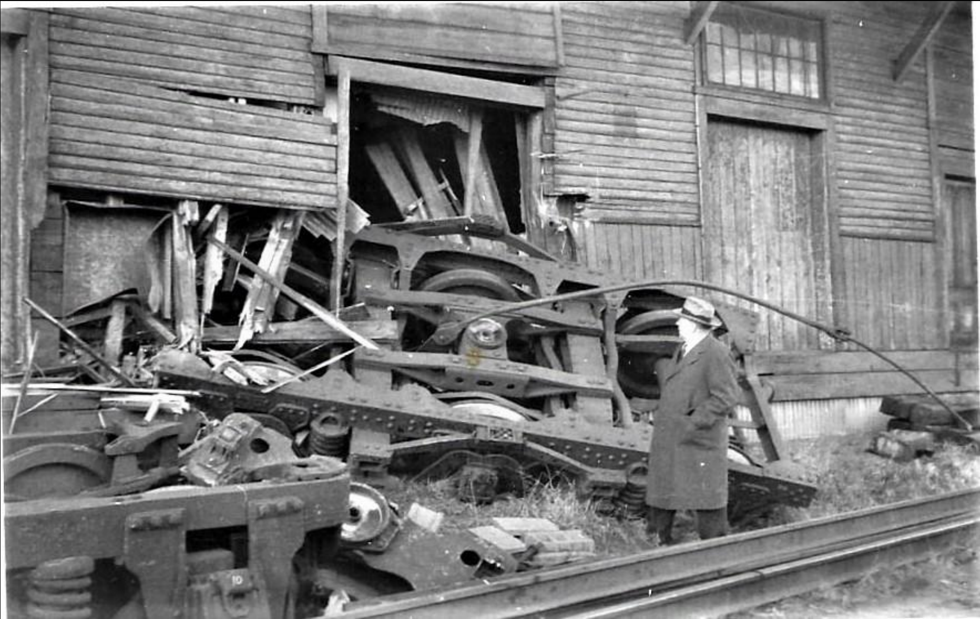
Passenger Trucks derailed into the Freight Shed
