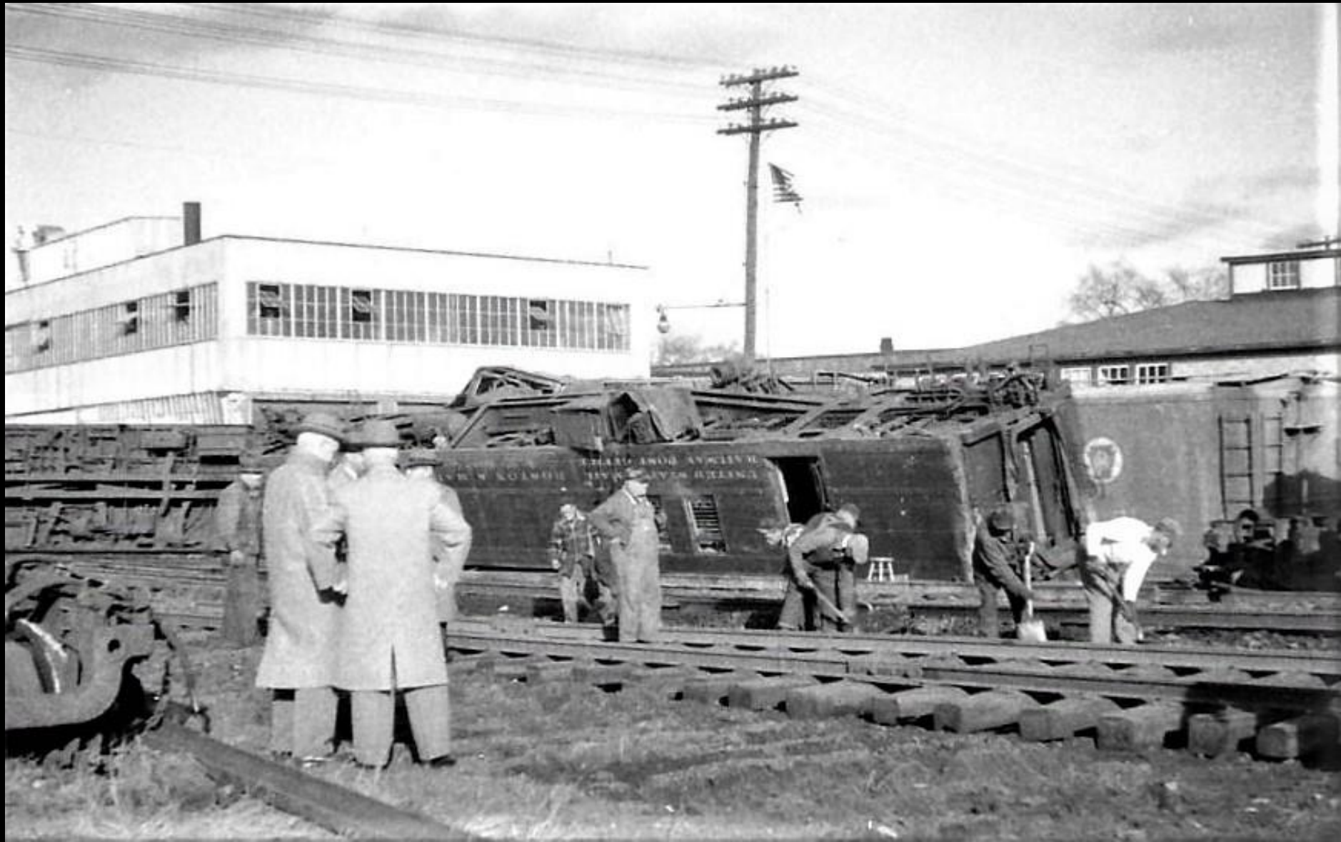
Boston & Maine Railroad R.P.O. #3100 landed on it's roof..
