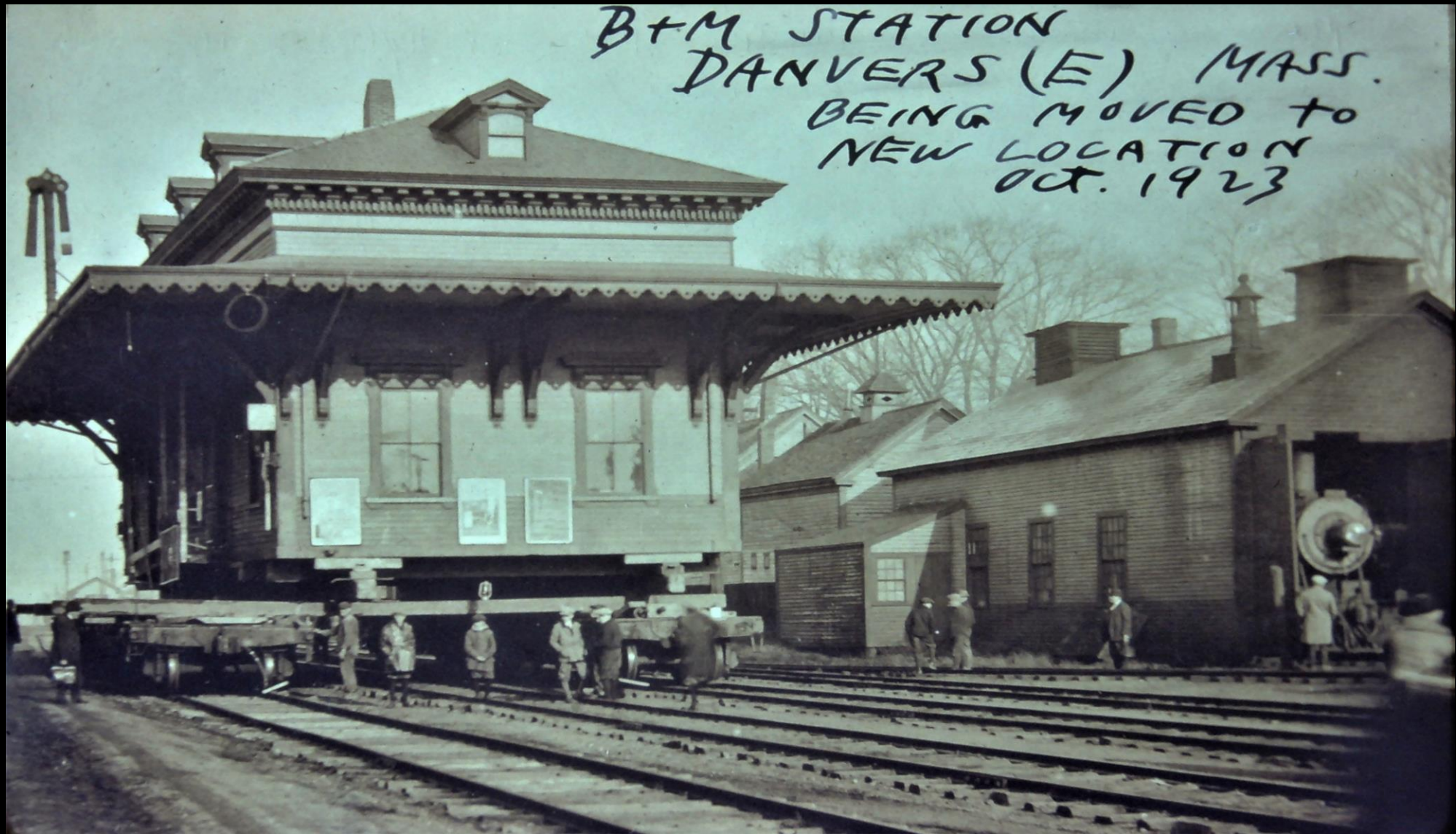
View of Danvers Station being moved Oct 1923
