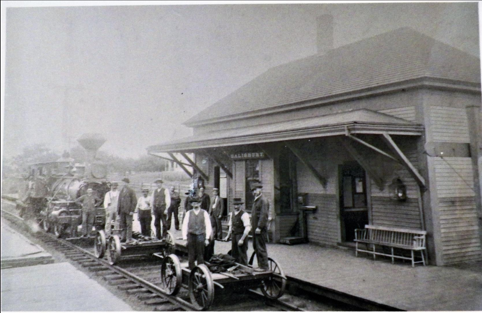
East Salisbury Station – Circa 1890 Track Gang with push cars & Steam Locomotive Push cars move material to the work site.
