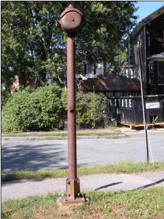
This rusty structure was in fact once the bell for the crossing of the Lexington Branch at Linwood Street in Arlington. Last used in the early 1980's, the structure was still standing the last time I rode my bike past this location. Andrew Riedl photo, 9/13/2009.
