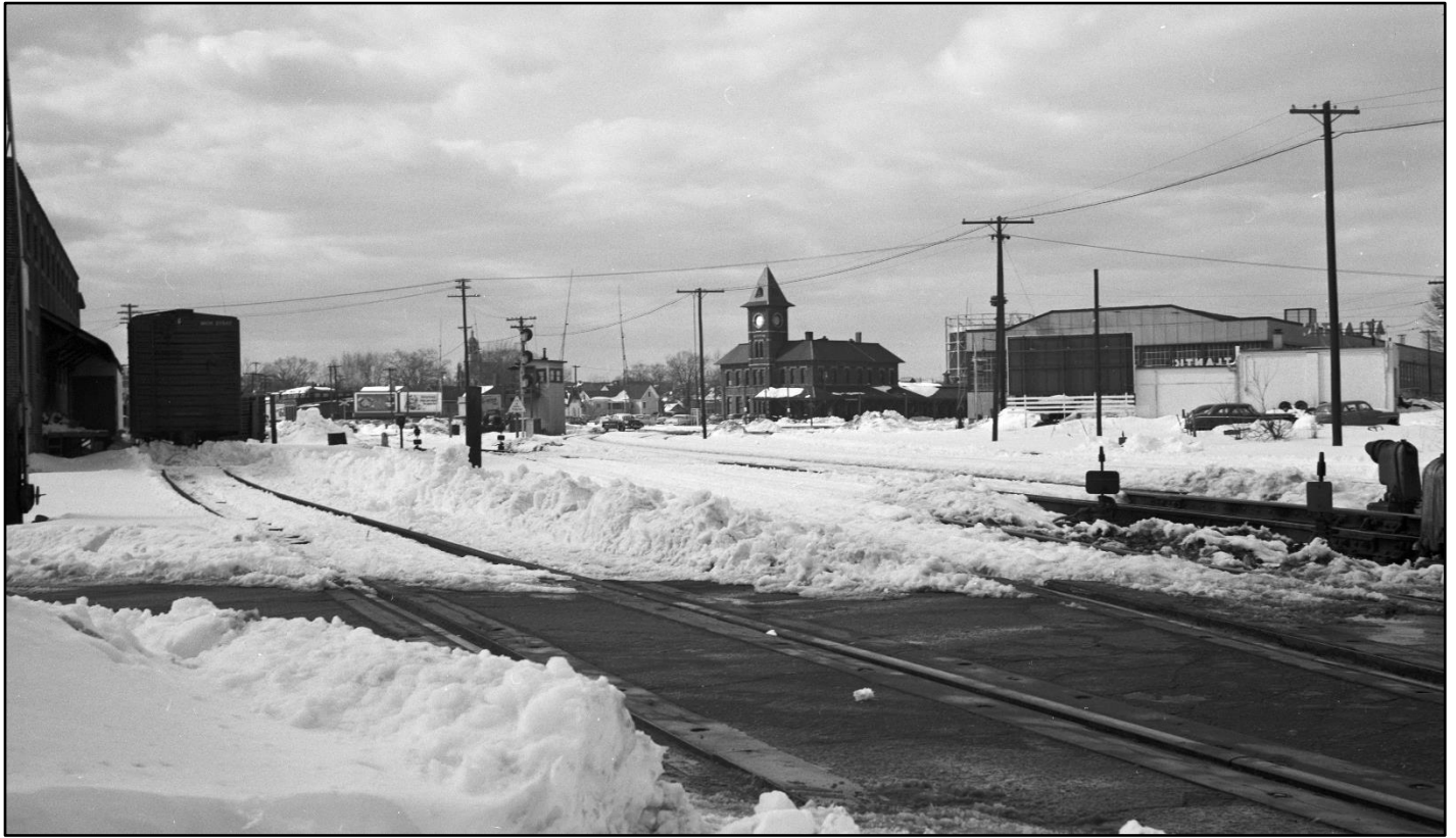
Above: Looking north at Crown Street in Nashua, NH on a winter's day in the late 1950s. The track at right is the New Hampshire Division Mainline which curves off to the right towards Nashua Union Station. The switch there is for the Hillsboro Branch, which heads off to the left of the image. Also visible are the crossing tower and gates for East Hollis Street, and a boxcar spotted at the LAW Warehouse. Nashua was a busy place then, with action not only in the yard and on the NH Division Mainline but also on the Hillsboro Branch. There were even numerous freight customers on stub-ended remnants of the Nashua, Acton & Boston and the Worcester, Nashua & Portland lines. Official B&M Railroad photograph, MacMillan/Hutchinson Collection, B&MRRS Archives.
