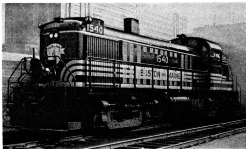
1600 H.P. Diesel for Local Passenger and Freight Service
