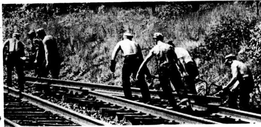
Cutting over to single track, Reed's Ferry, N. H.
