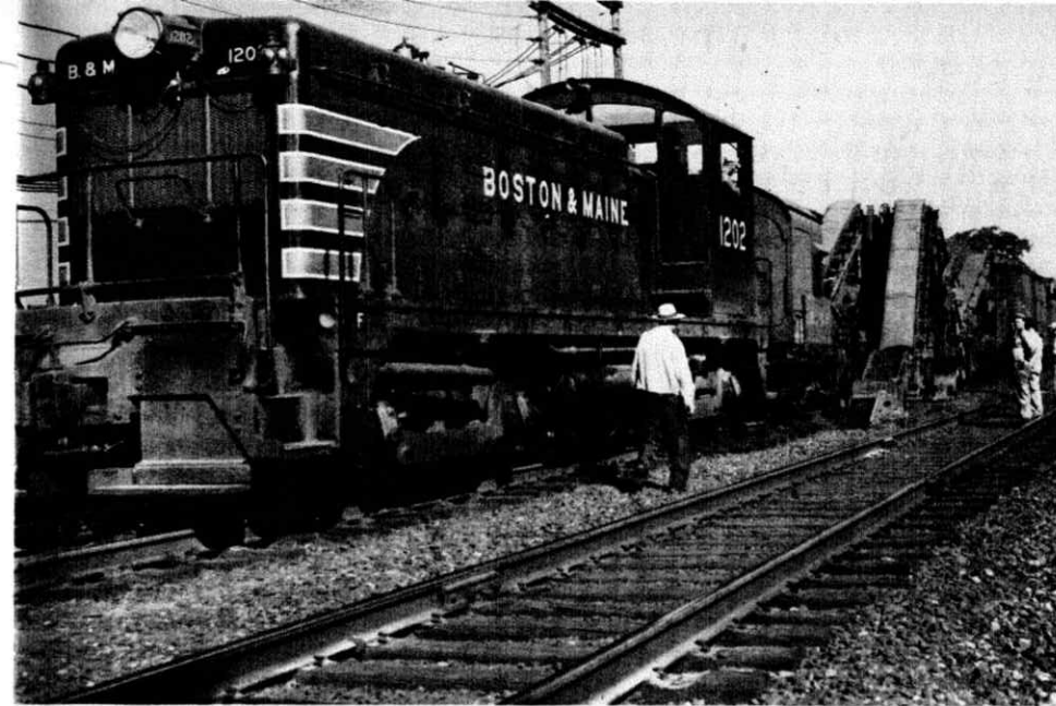
(Above) Cleaning ballast on the Boston and Maine. The ballast is picked up, the dirt sifted out and the ballast replaced in the road bed. (Below). Another view showing the dirt from ballast being expelled to one side
